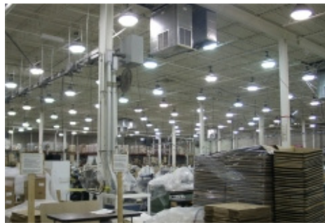
Photo Top: Metal Halide Lighting
